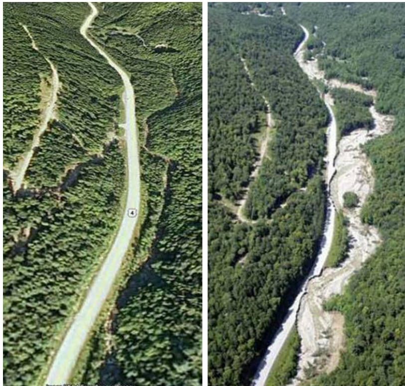
Route 4 Before and After Tropical Storm Irene | Source: USDA Farm Service, Google Earth
